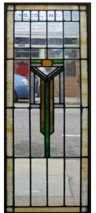
Stained Glass Repair Cabinet Door Compton, CA, 2007
